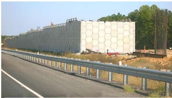
Figure 1: Typical use of MSE walls as bridge abutments
